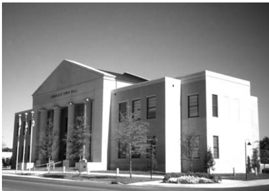
Figure 11.4 Cornelius Town Hall, Shook Kelley Architects, 1999. The monumental scale of the new town hall was a shock to many local residents, used to paying their taxes and going to meetings in a single-storey shed for several decades. While this building works well and provides excellent facilities for the town, the authors can’t help but wish the architecture had made a more contemporary statement rather than retreating into historicism.
